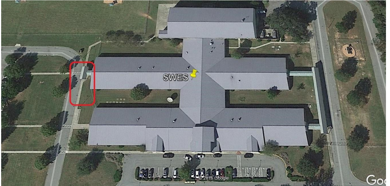
SCHOOL SITE WITH CANOPY LOCATION IDENTIFIED
